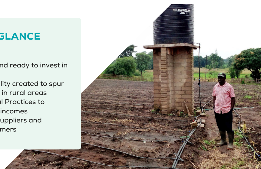
Small-scale solar irrigation systems installation/E4I
